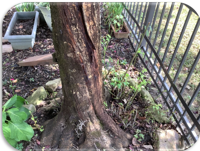
Look for cracking
